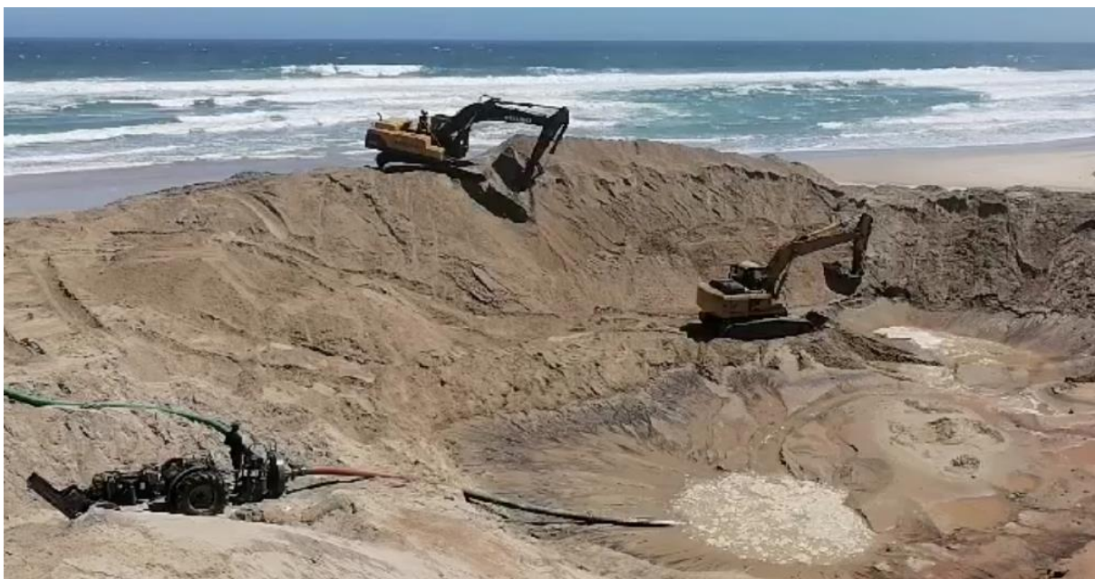
Photo 1: Berm to prevent waves from entering excavation
