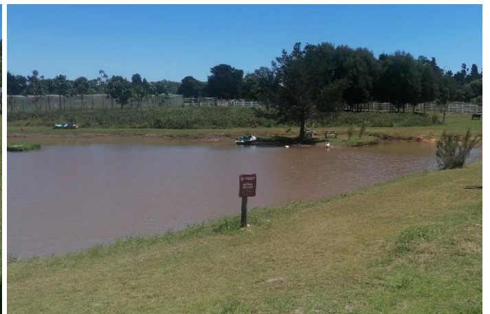
Photo 4: Recreational Dam – Dam No. 3
