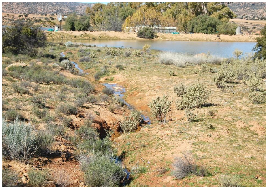
Figure 13 Redirected flow into the farm dam
