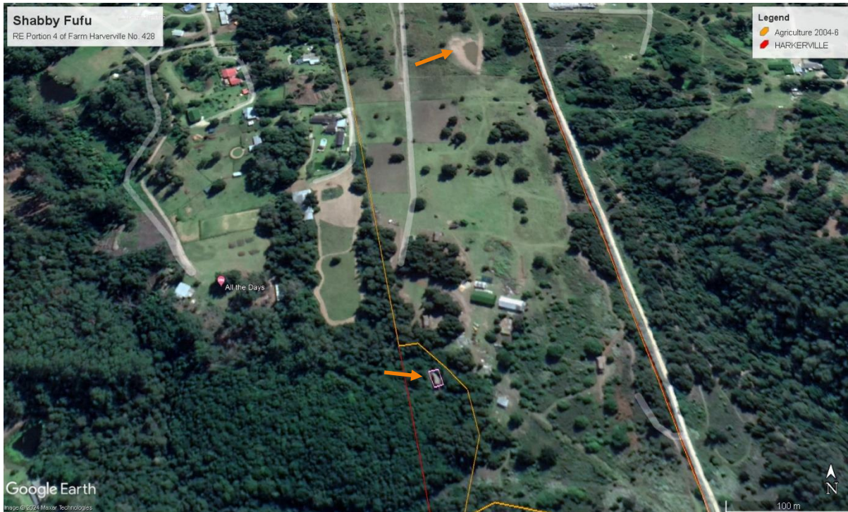
Figure 7: Google Image (May 2018) showing the construction of the dam and one small cottage outside of the original disturbance footprint (pink).
