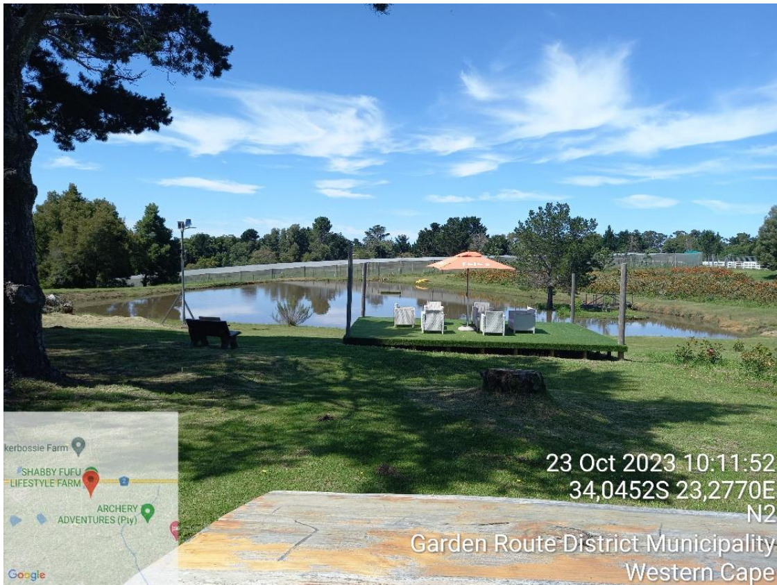
Photograph 2: View of the dam constructed within a watercourse.
