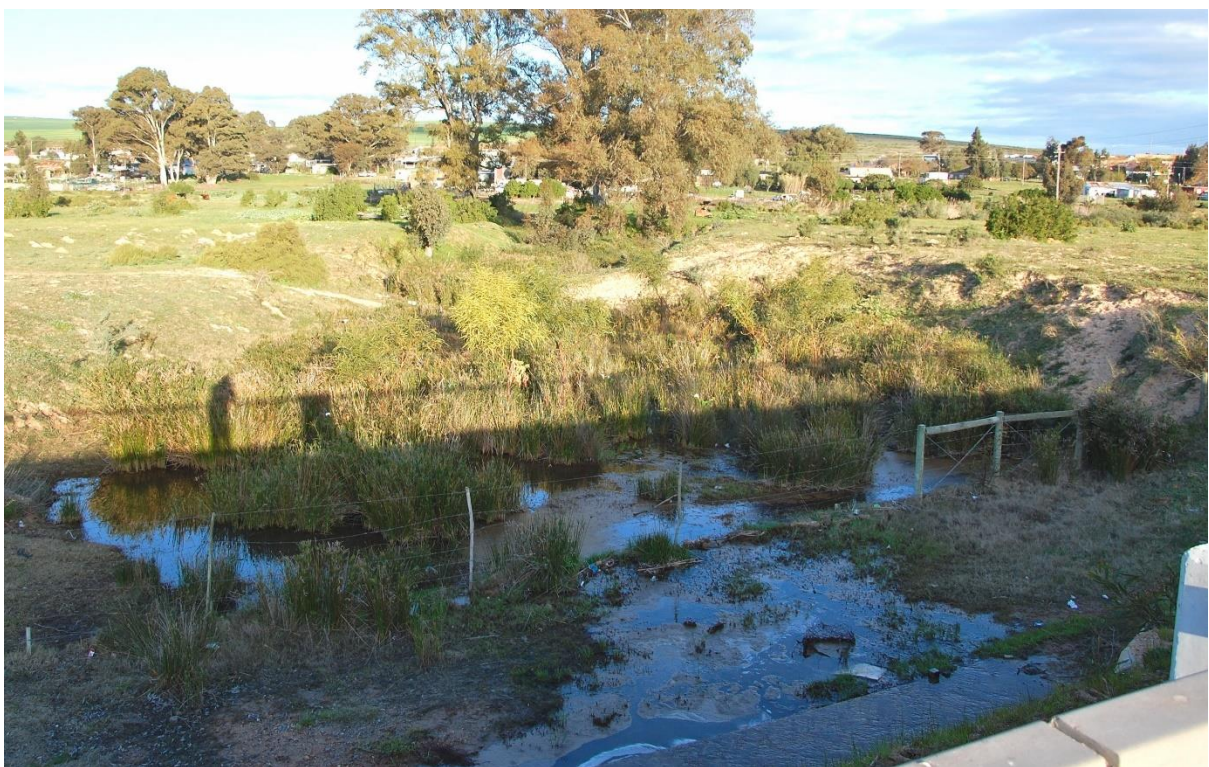
Figure 11 Drainage line No.2
