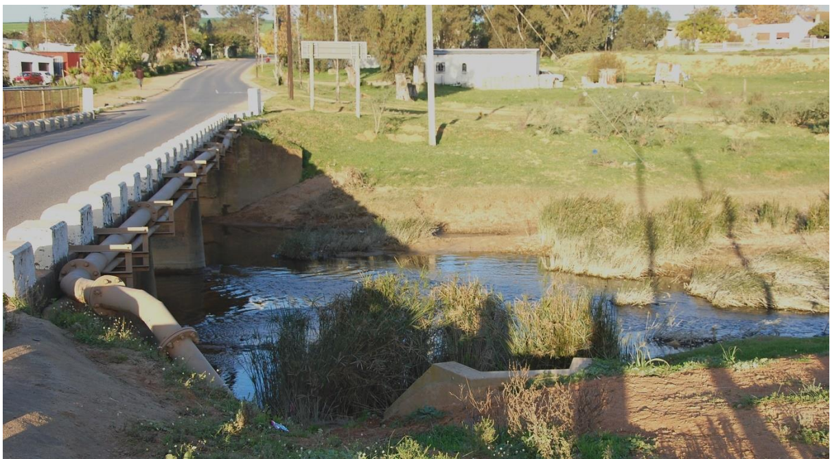
Figure 13 Bloemendal Road bridge
