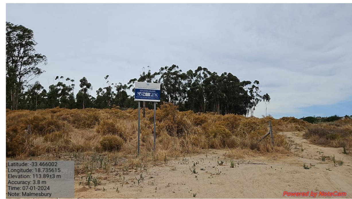
Photograph 20: Klipkoppie Solar PV facility Road View 8
