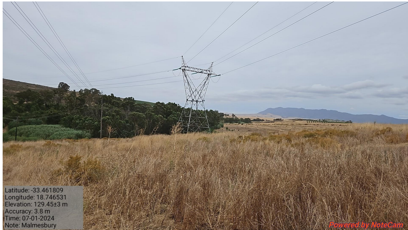
Photograph 1: Existing Medium Voltage OHLs surrounding the Klipkoppie Solar PV facility Development Area
