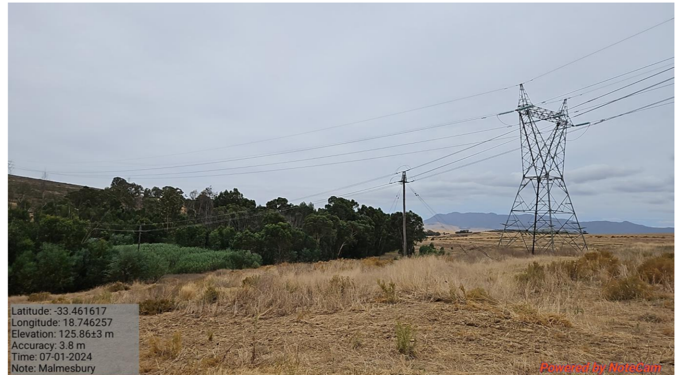
Photograph 10: Existing OHLs within the Klipkoppie Solar PV facility Development Area
