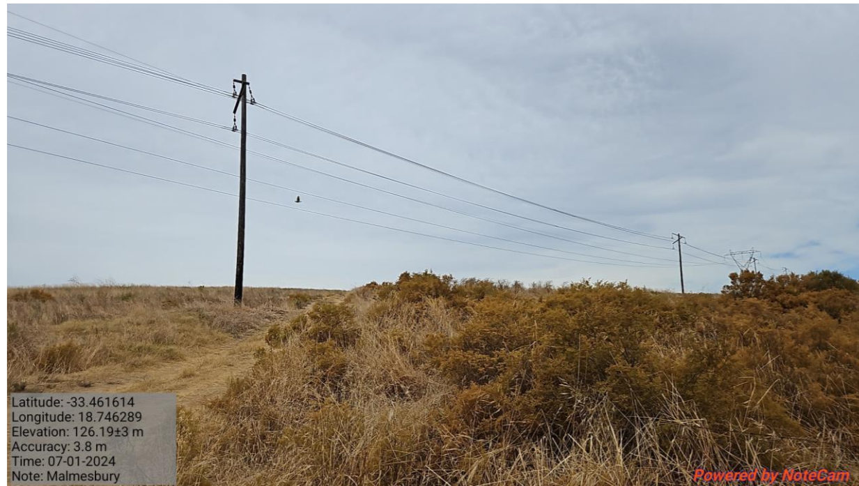
Photograph 13: Klipkoppie Solar PV facility Road View 1
