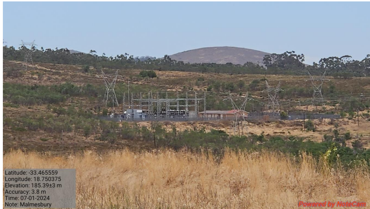
Photograph 9: Existing Substation near the Klipkoppie Solar PV facility Development Area
