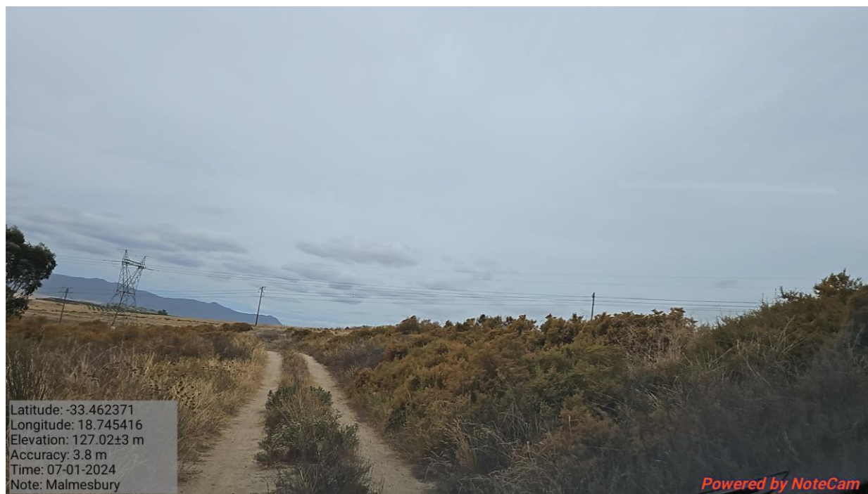
Photograph 15: Klipkoppie Solar PV facility Road View 3
