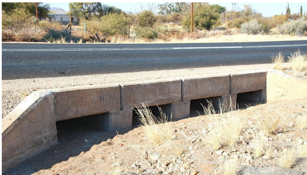
Figure 16 Constructed box culverts.
