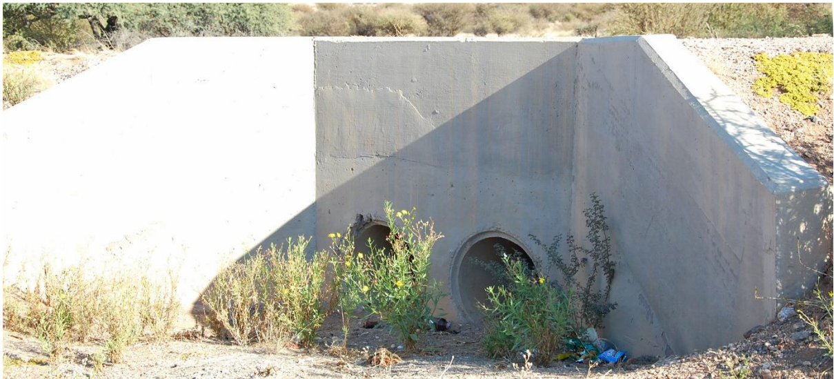
Figure 9 N14 road bridges
