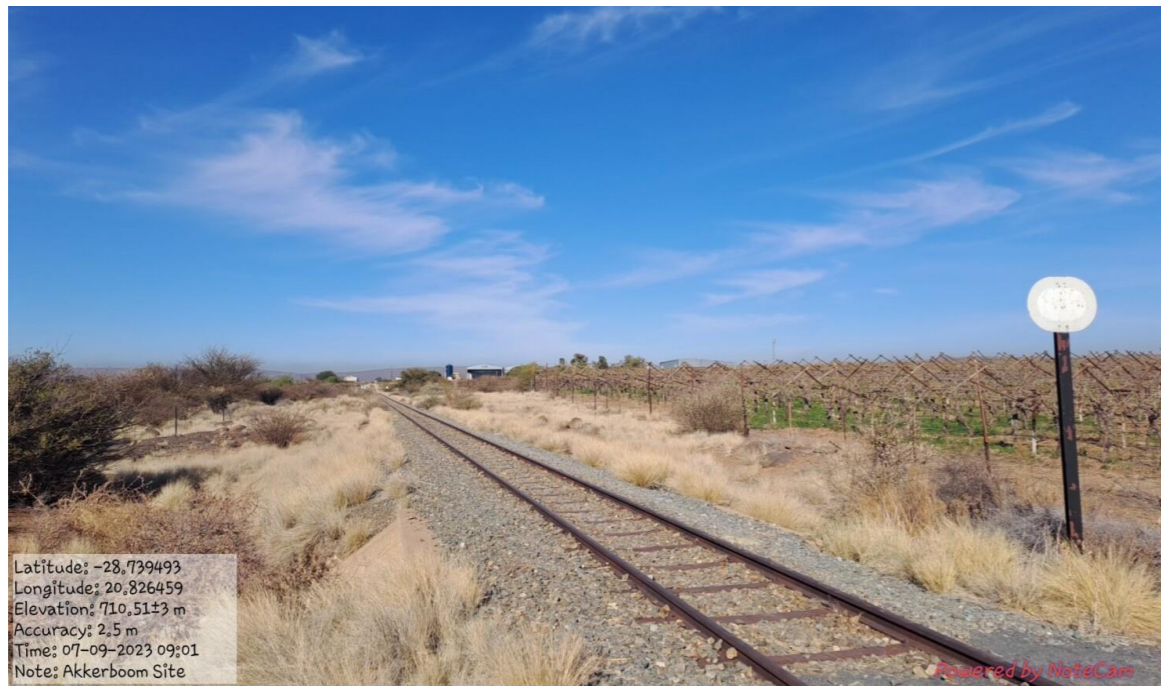
Photograph 15: Railway Tracks Parallel to the Development Area
