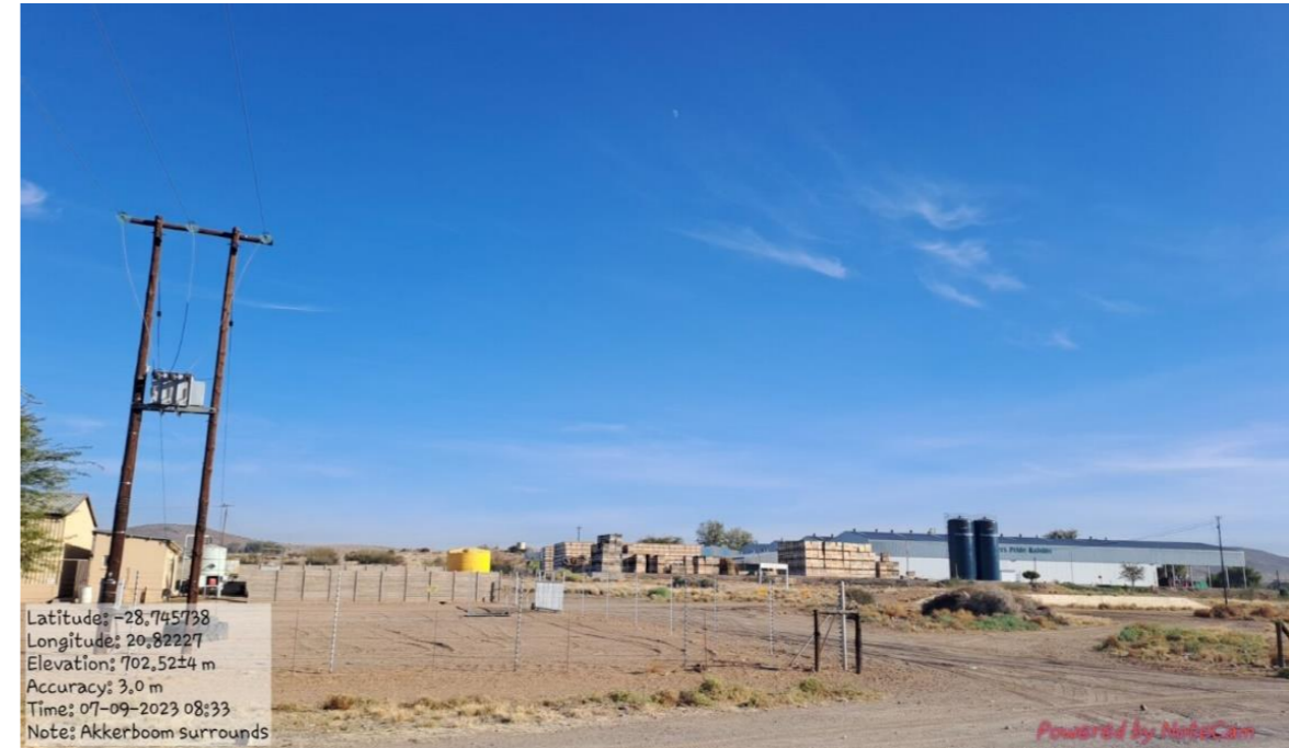
Photograph 6: Industrail Businesses on Neighbouring Properties of the Proposed Development Area.
