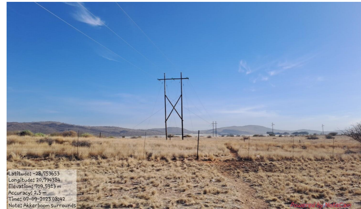
Photograph 2: Example of Electrical Infrastructure within the Development Area
