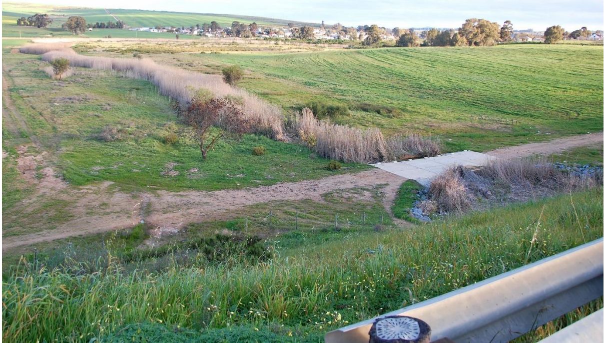
Figure 10 Drainage line No.1
