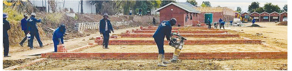
Construction workers hard at work at the proposed new industrial hub.
