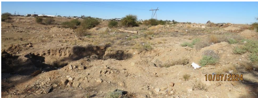
Photo 3: View of existing excavations that form part of site disturbance
