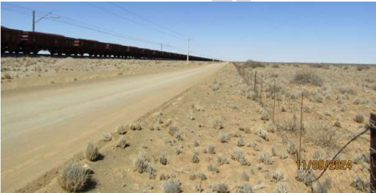
Photo 12: Disturbed roadside of the Sishen-Saldanha railway servitude
