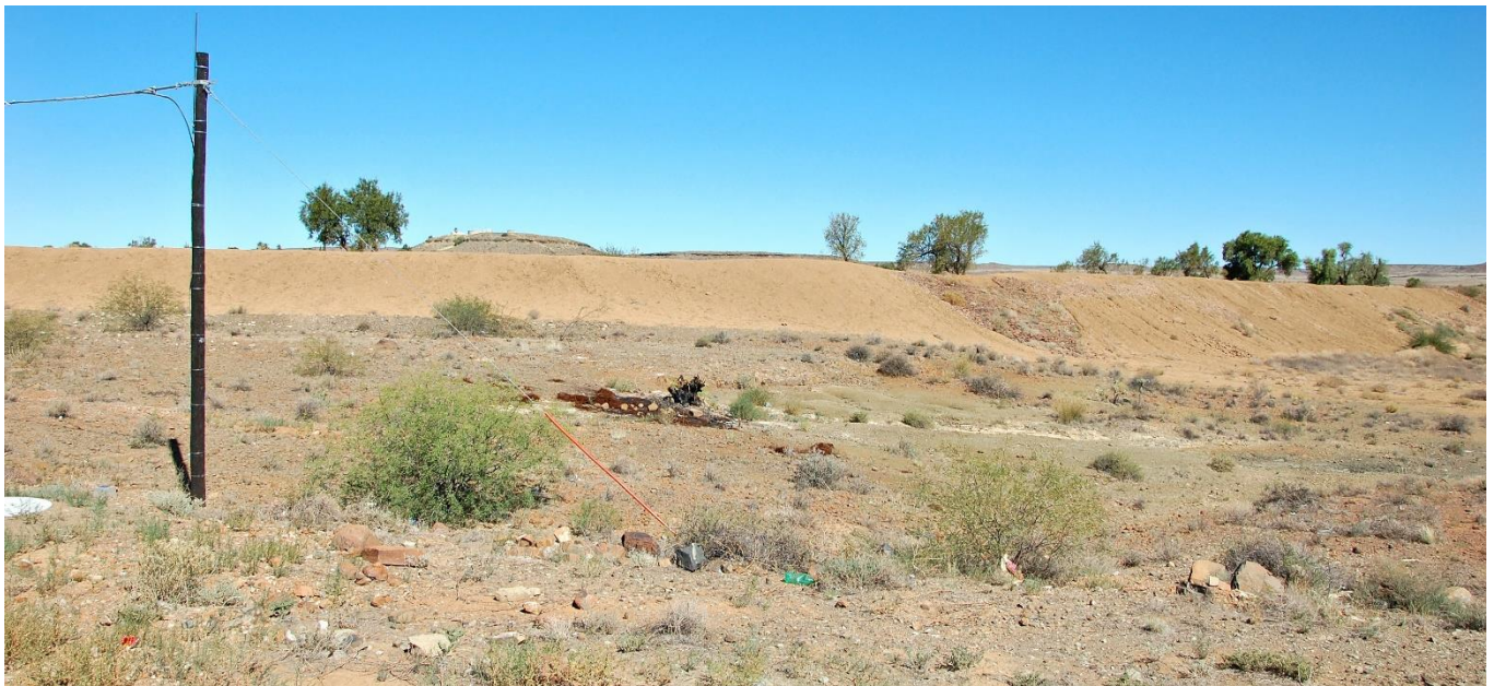
Figure 12 Western dam wall
