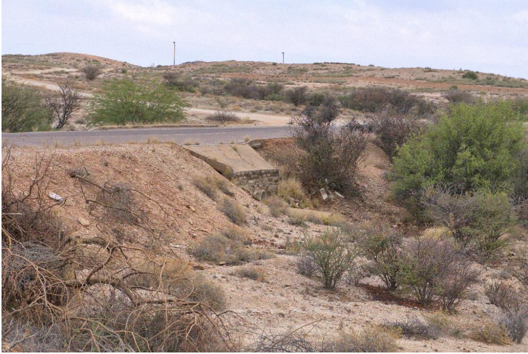
Figure 13 Storm water pipes
