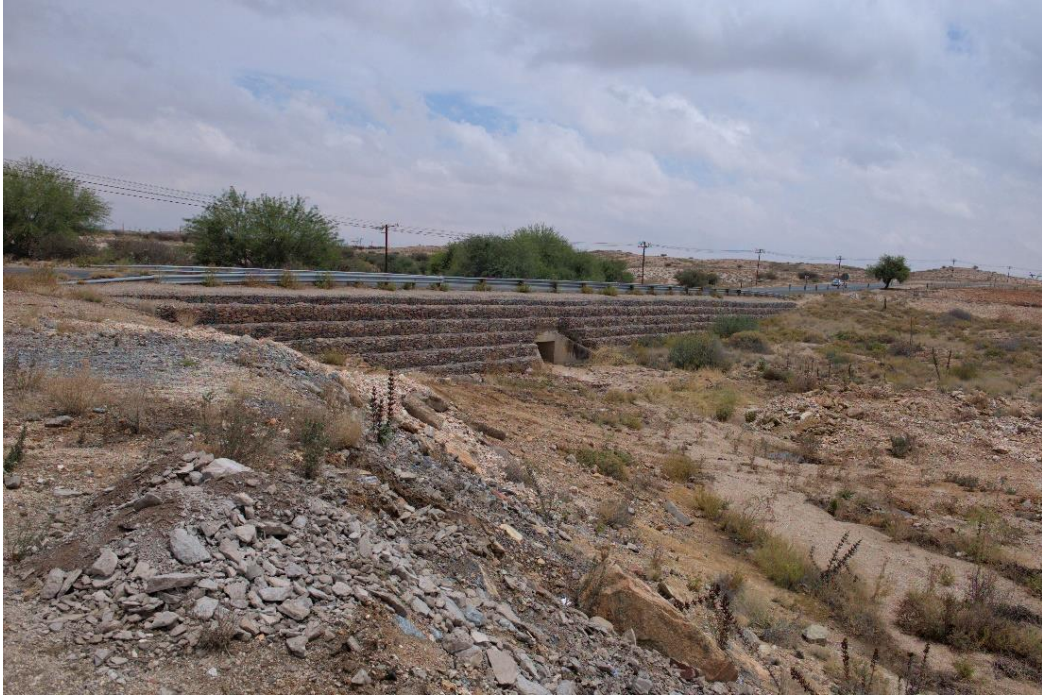
Figure 9 N14 Embankment and culvert
