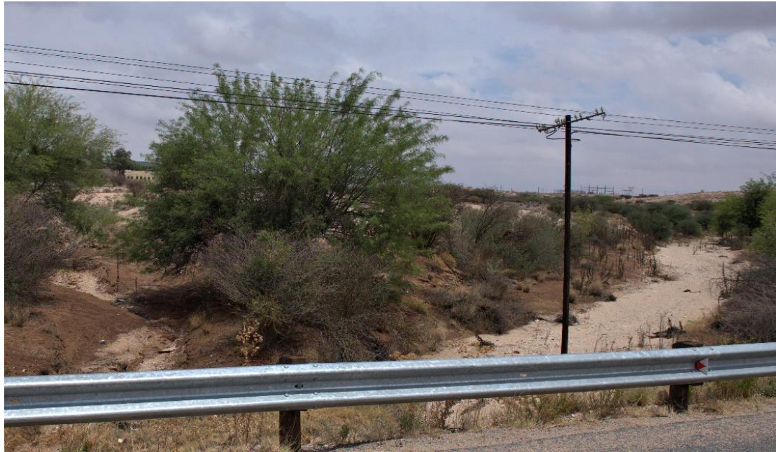
Figure 11 Drainage line upstream of N14 culvert
