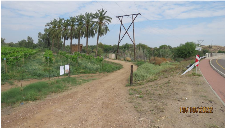
Photo 1: Looking from east to west onto the existing pump house for the Kenhardt pipeline. Note the disturbed nature of the area and agricultural land to the left of picture.
