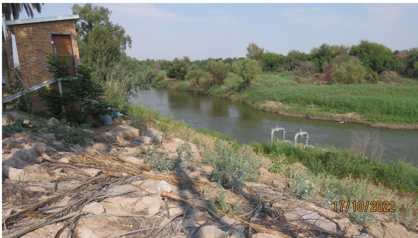
Photo 2: The existing pump house, next to which the new pump house will be located. Note the existing disturbance footprint.
