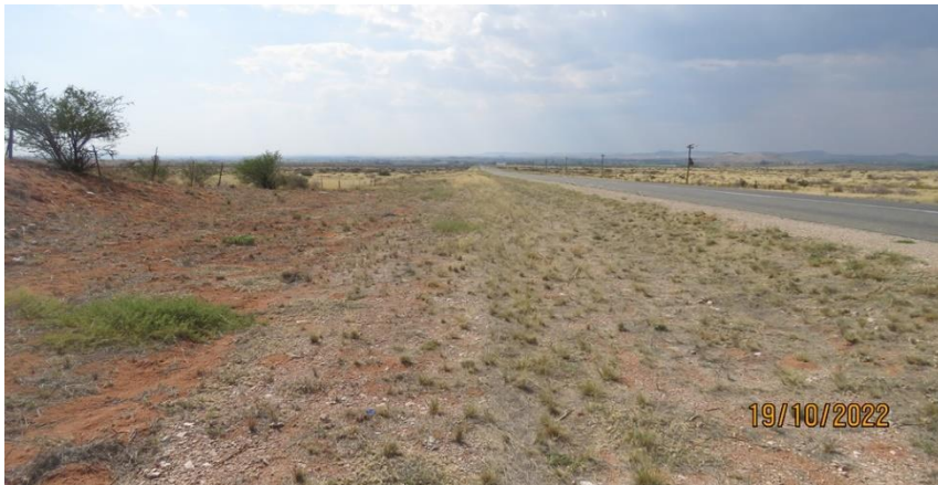
Photo 11: Looking from south to north back towards Lennertsville, showing the typical status of the road reserve. Note the low vegetation height and clear indications of brush cutting.
