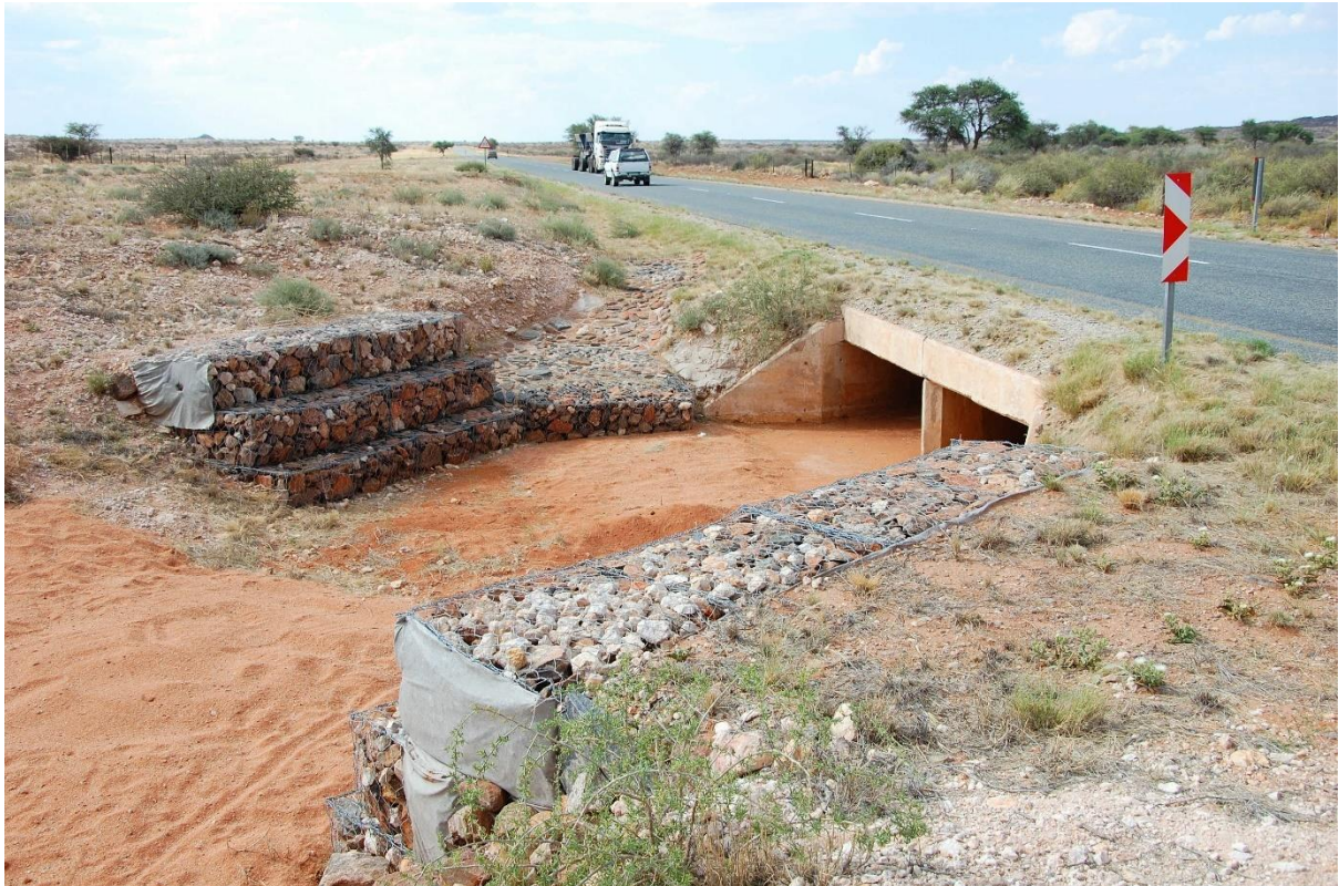
Figure 21 Continued Point No.7 drainage line crossing
