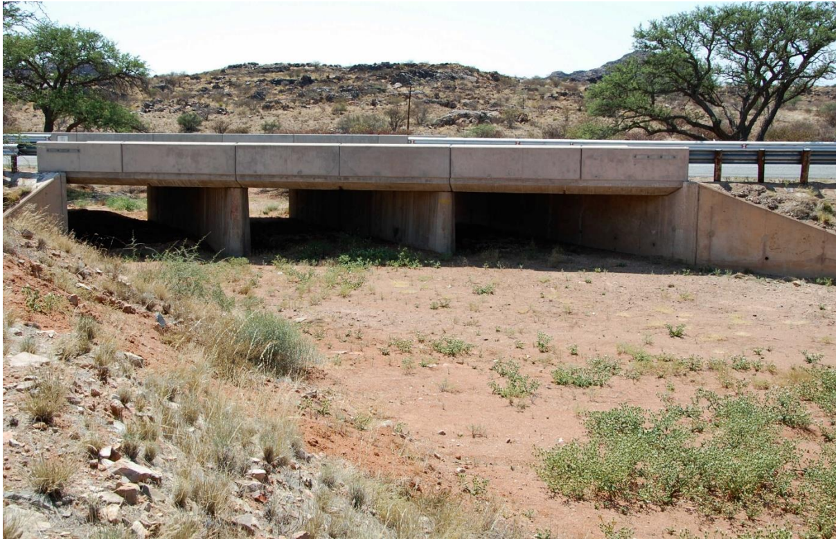
Figure 18 Bridge at Point No.6
