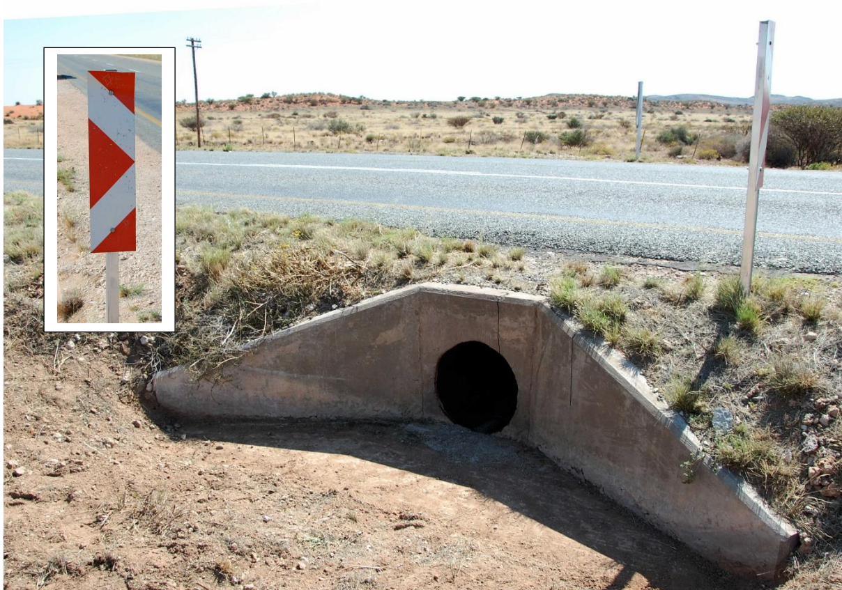
Figure 9 Class 1 drainage line with pipe culvert.
