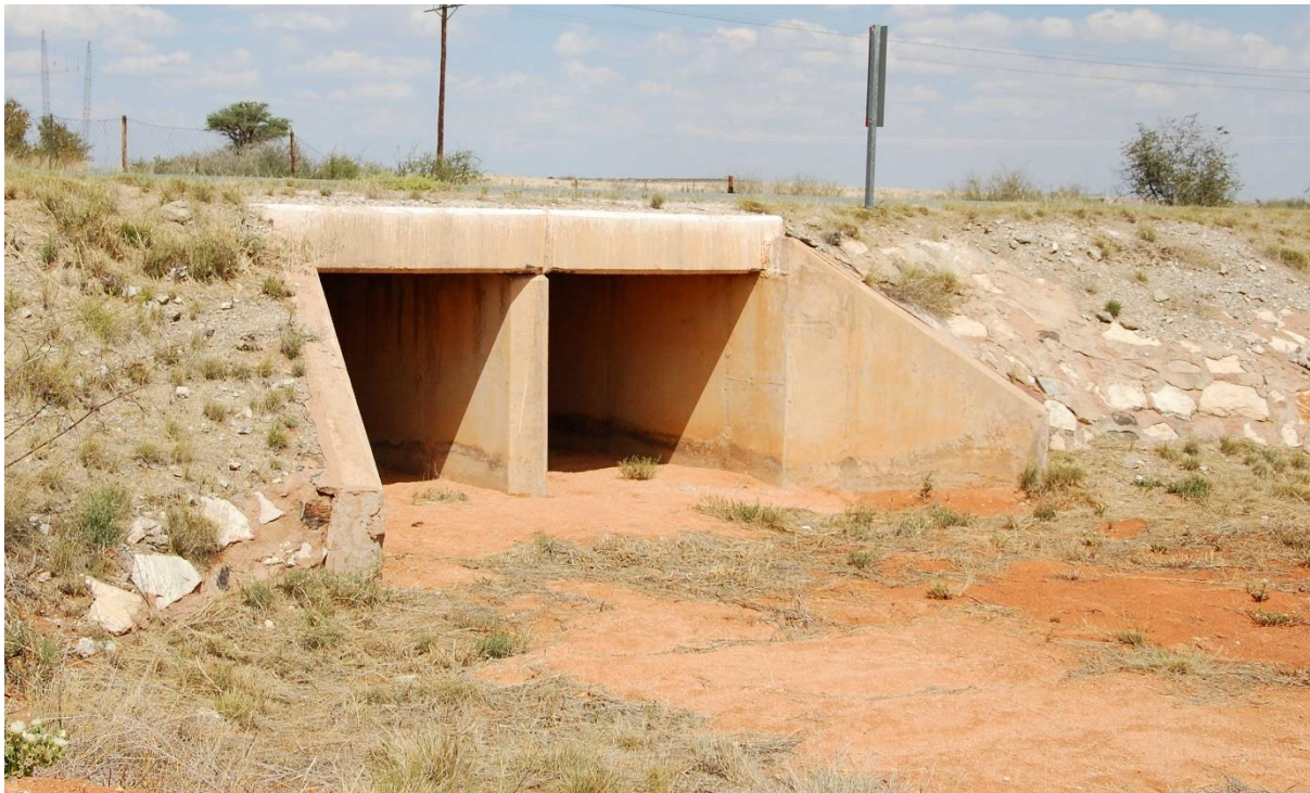
Figure 26 Culverts at Point No.12.
