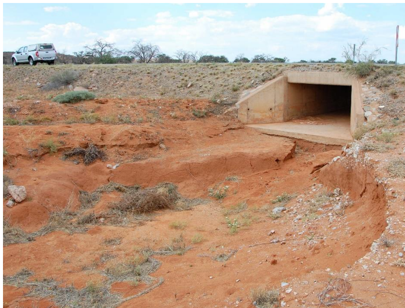
Figure 23 Point No.9 Box culverts
