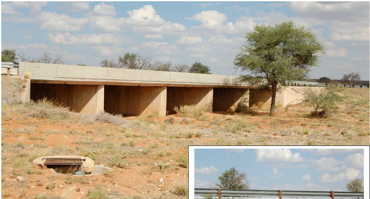
Figure 22 Bridge and box culvert at Point No.8 crossing
