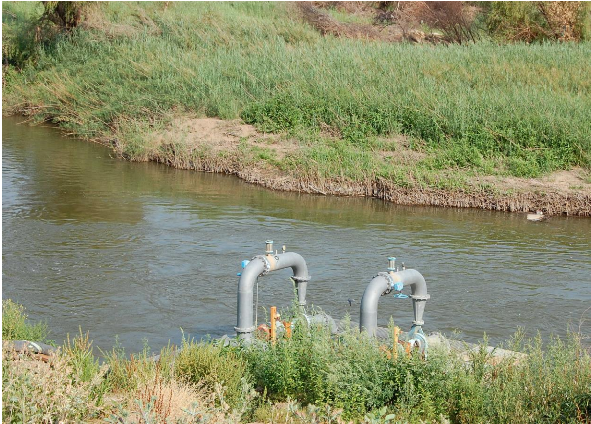
Figure 11 Raft and pumps
