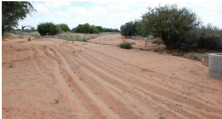
Figure 25 Culverts at Point No. 11
