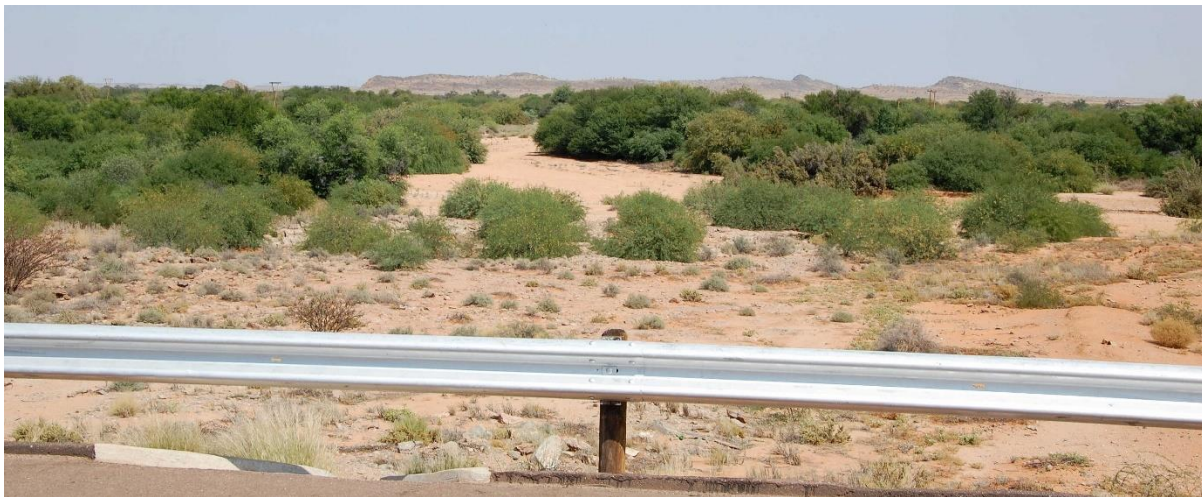
Figure 29 R27 Road bridge south of Kenhardt
