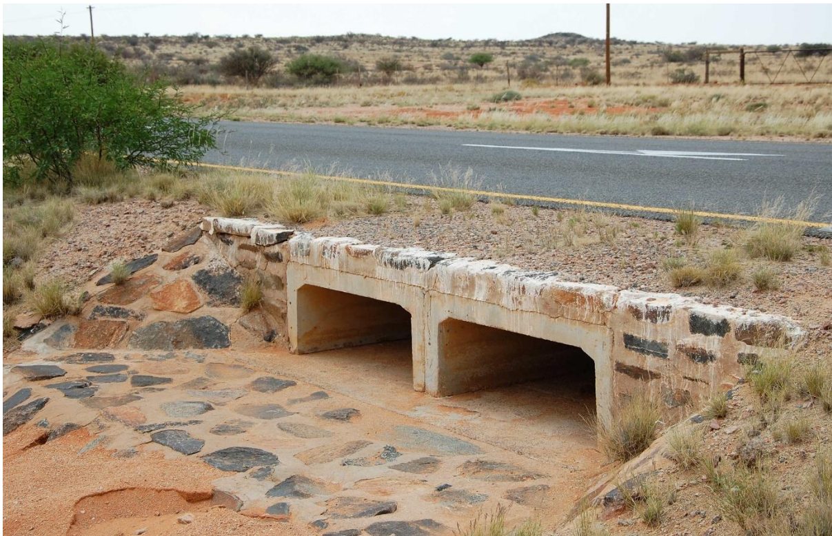
Figure 40 Culvert at Point No. 23
