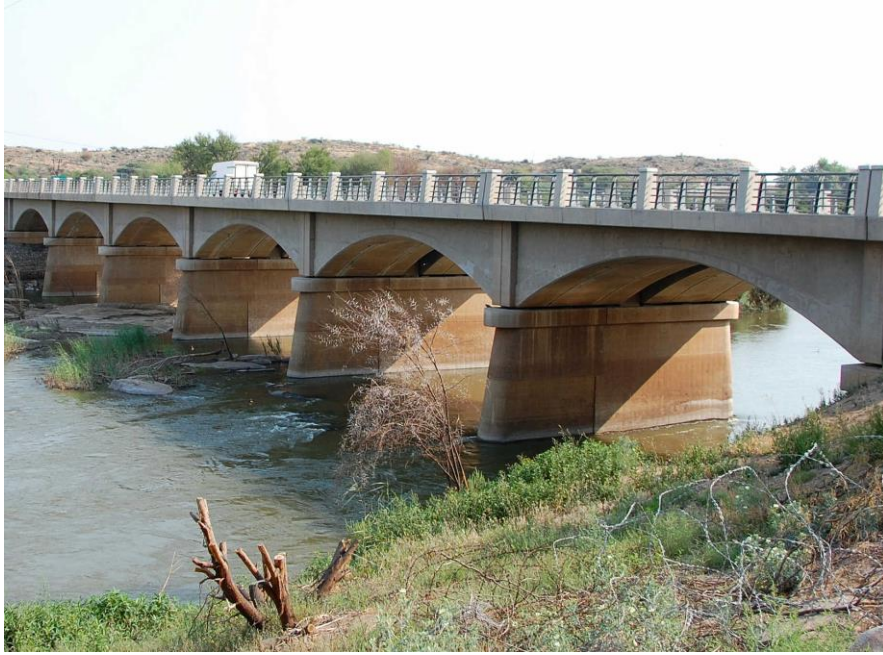
Figure 54 R27 Road Bridge
