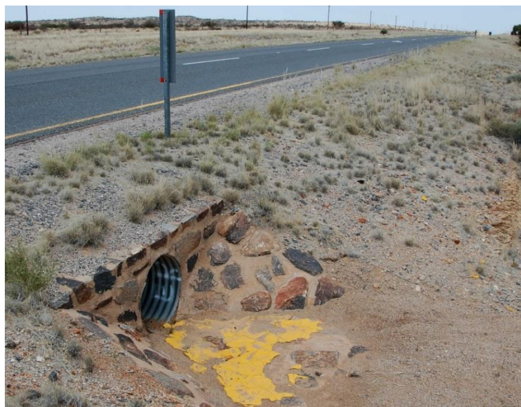
Figure 38 Pipe culvert at Point 20
