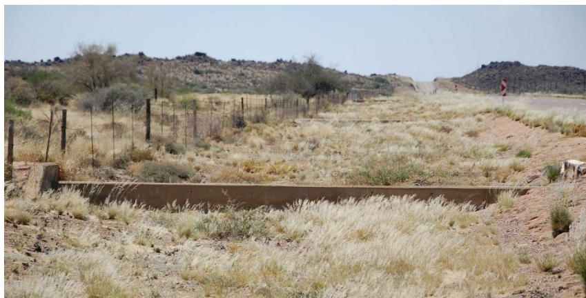
Figure 57 Flood control walls
