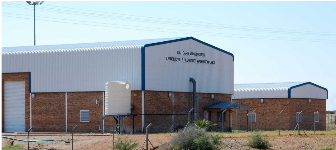
Figure 15 Crossing at Point No.2 at municipal water works.
