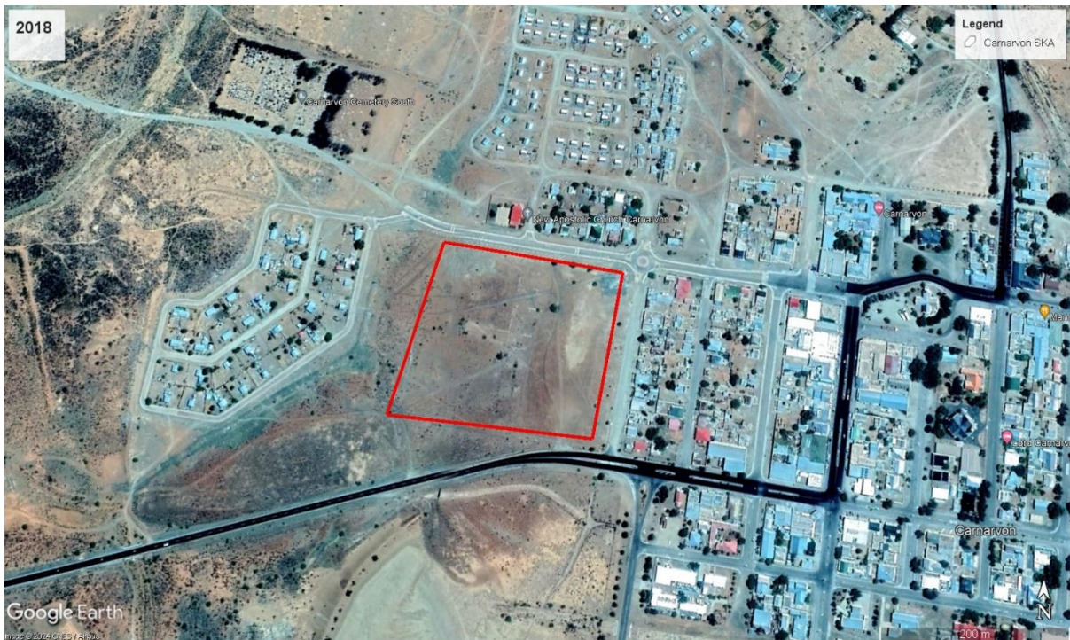
FIGURE 16: GOOGLE SATELLITE IMAGE OF THE CARNARVON DEVELOPMENT SITE (2018).
