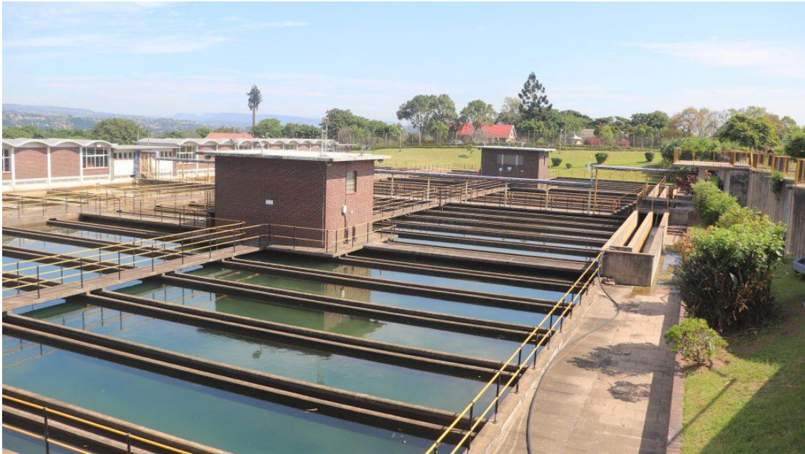
Figure 7: Umgeni Water: Raw Water Storage
