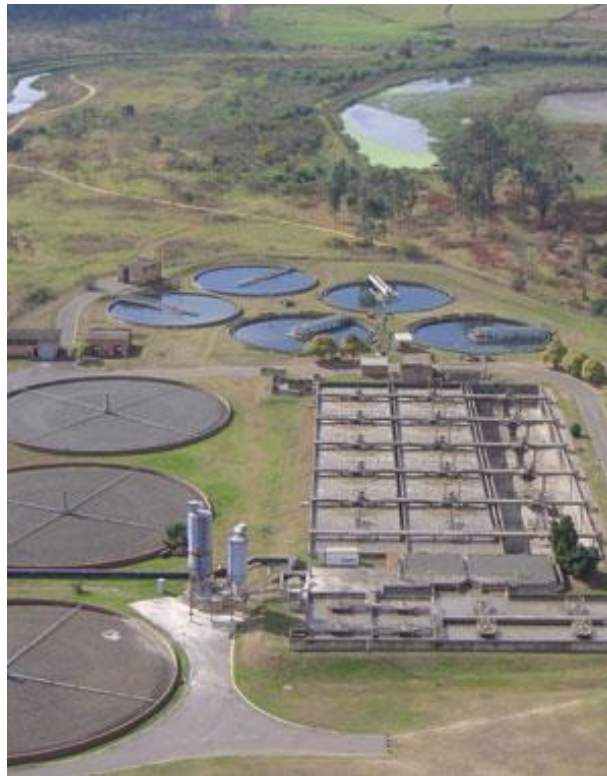
Figure 9: Waste Water Treatment Works: Umgeni Water: Darvill, Pietermaritzburg
