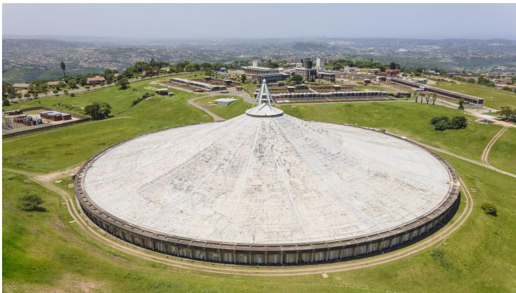
Figure 11: Durban Heights Reservoir 3
