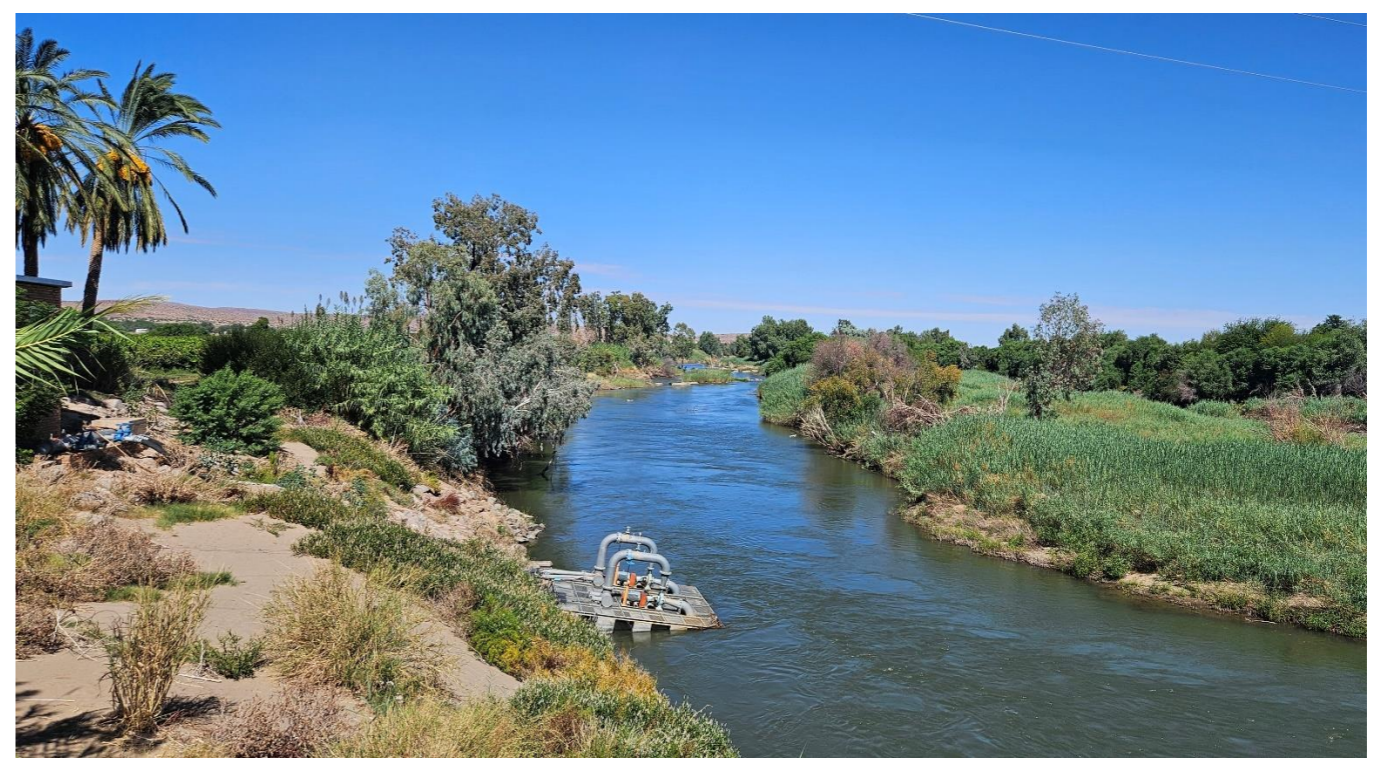
Photograph 8: Water Infrastructure along the Development Area.
