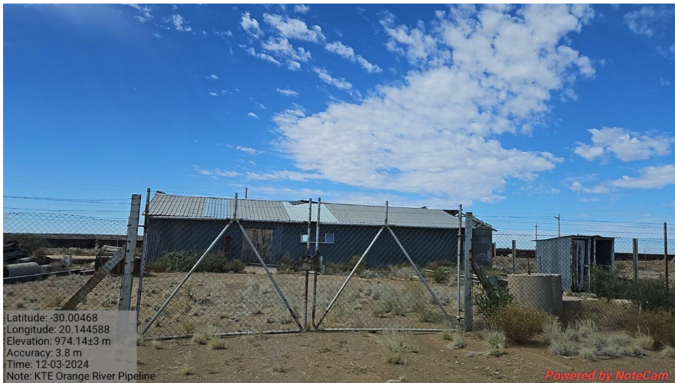
Photograph 7: Intact Infrastructure along the Proposed Development Area.
