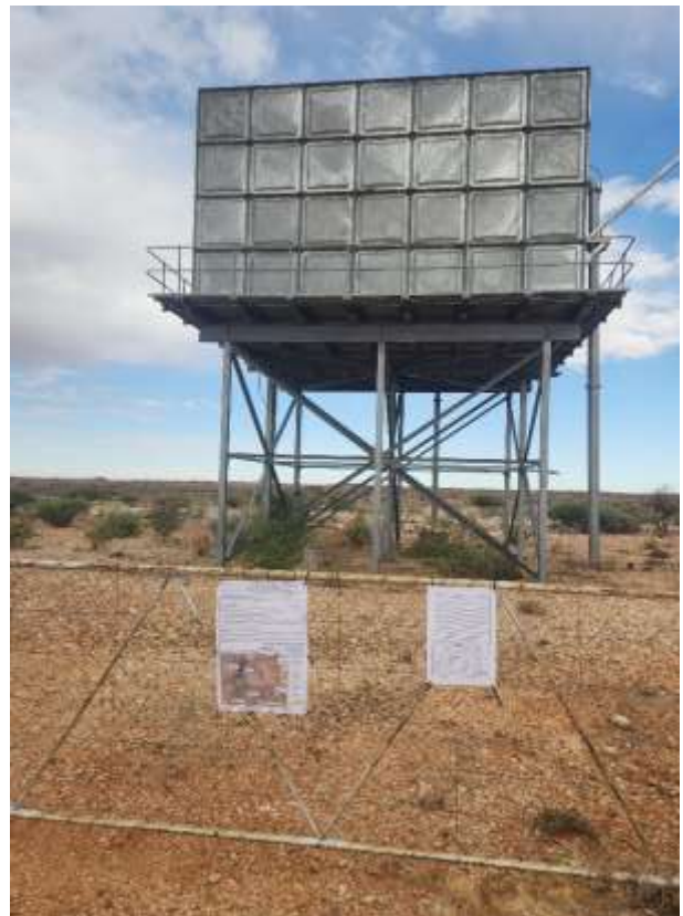
Photo 16: Proof of Site Notice placed at Piet Rooi Reservoir
