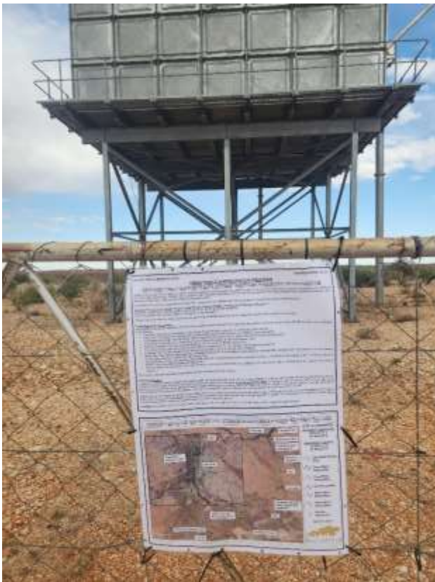
Photo 15: Proof of Site Notice placed at Piet Rooi Reservoir
