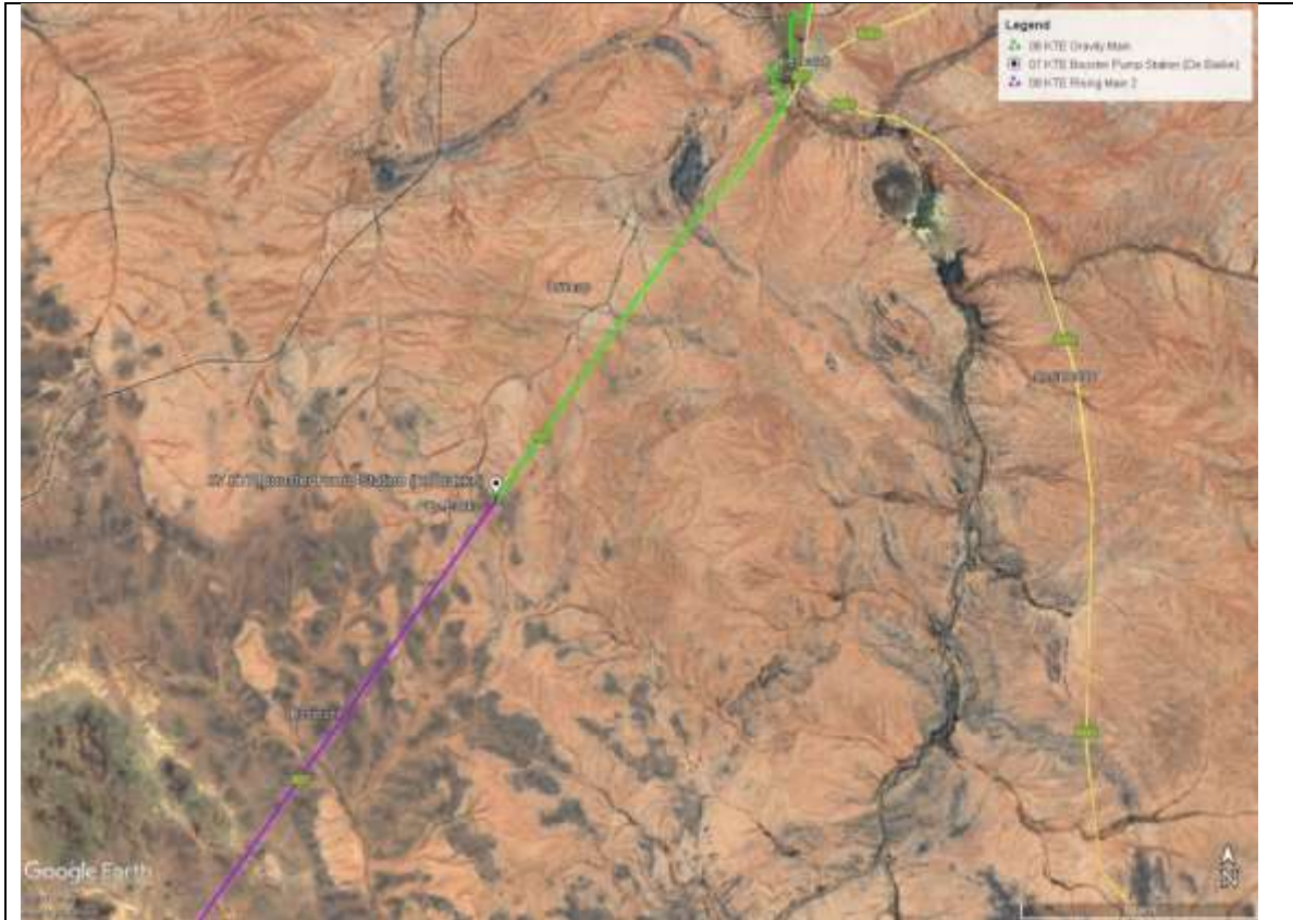
Figure 3. Close up view of the pipeline from Kenhardt to the De Bakke Booster Pumpstation.
