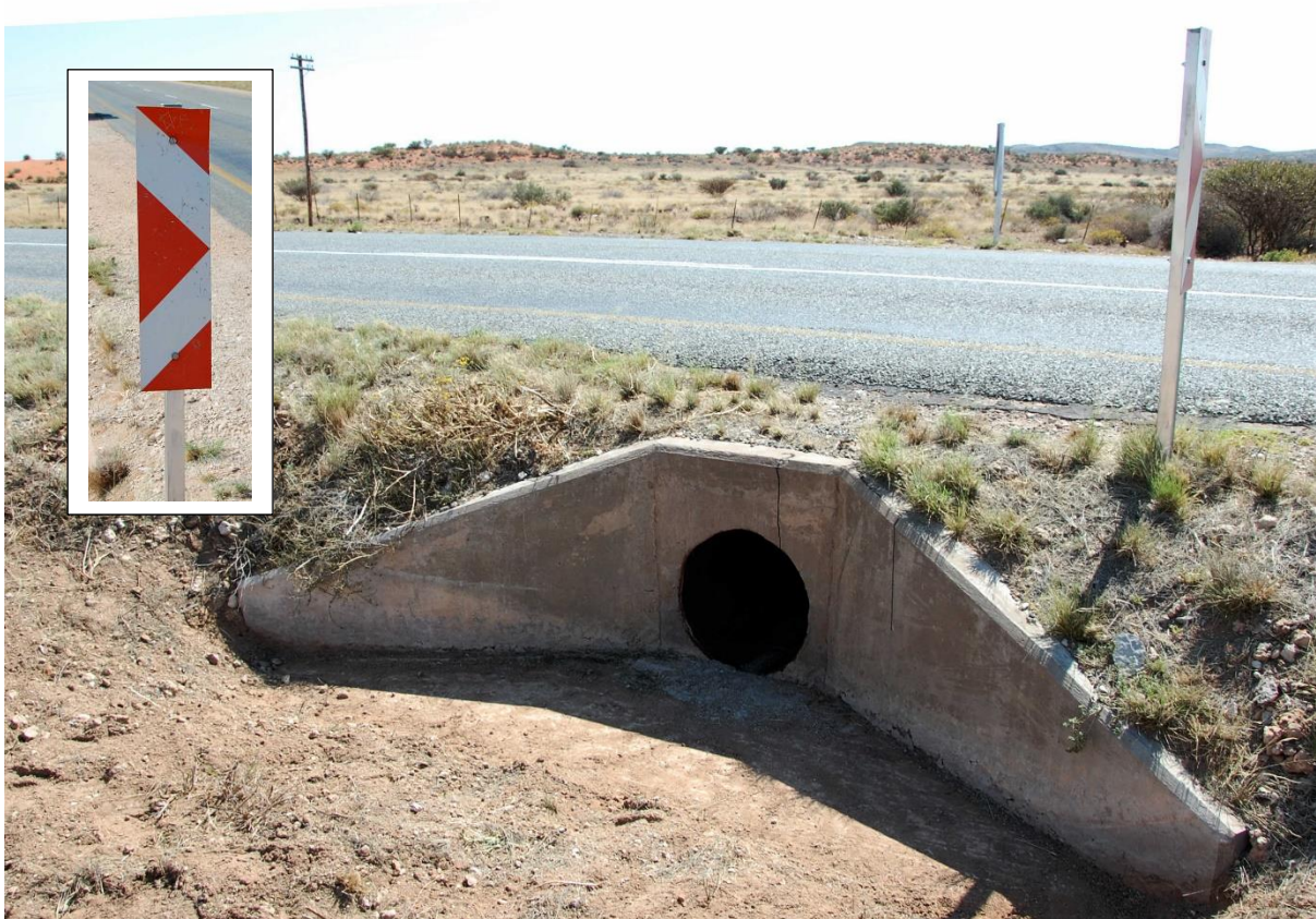
Figure 6 Class 1 drainage line with pipe culvert.
