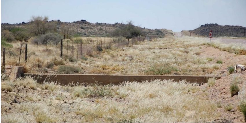
Figure 15 Flood control walls
