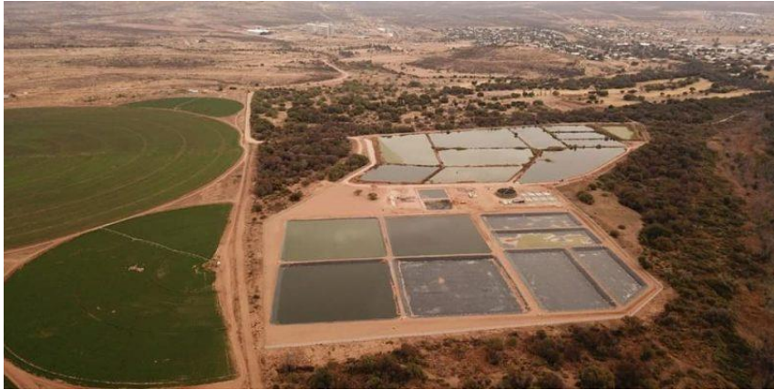
Figure 6: Prieska Wastewater Treatment Works, Northern Cape
