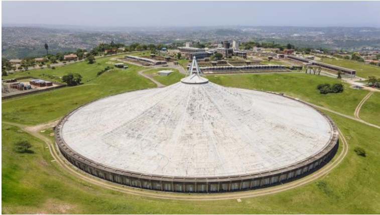
Figure 10: Example of a Reservoir
