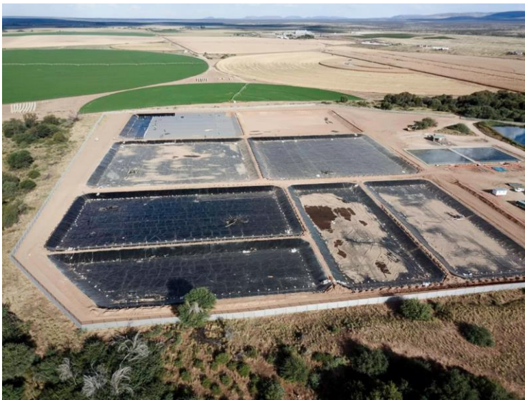
Figure 7: Prieska Wastewater Treatment Works, Northern Cape
