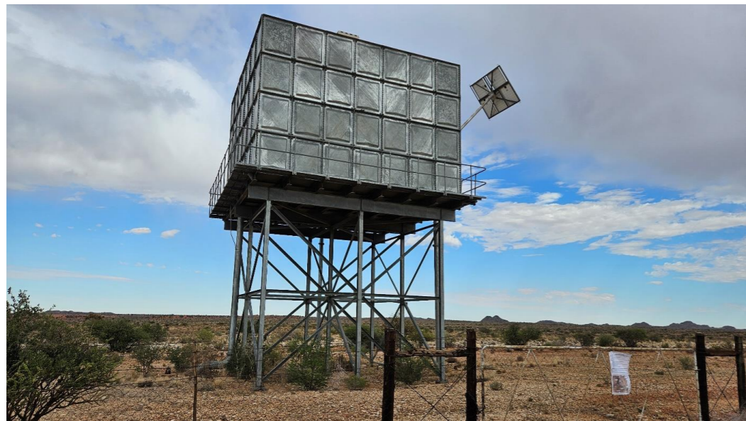
Photograph 3: Brandvlei Reservoir along the Development Site
