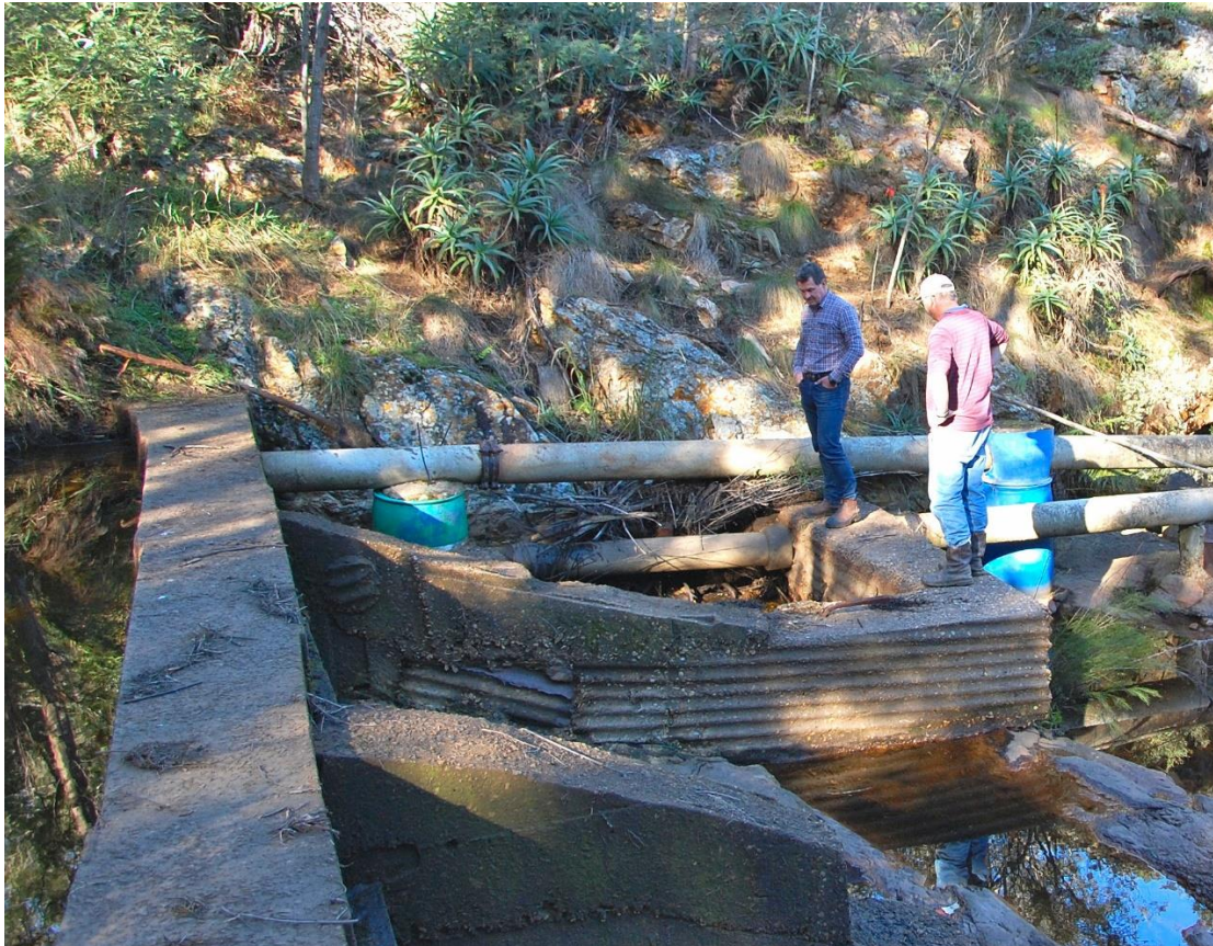
Figure 15 Weir and conduits in the middle Plattekloof River
