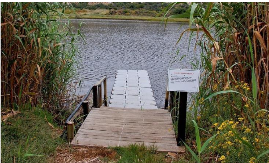
Photo 8: The small floating jetty at the Duivenhoks River. Note the minimum impact associated with the construction of the jetty (which could be easily removed and rehabilitated).
