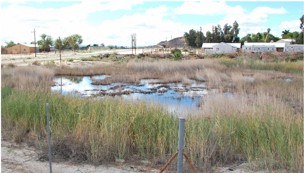
Figure 12 Runoff backing up against the street
