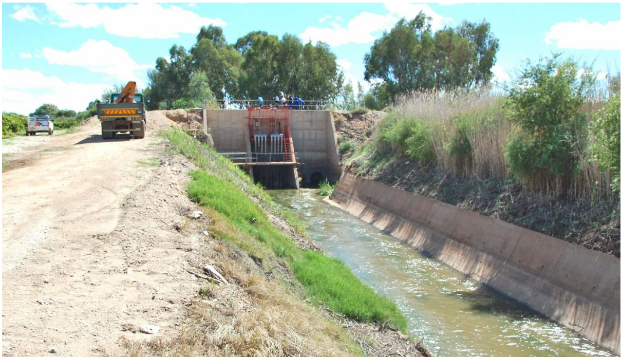
Figure 14 Sluice gate
