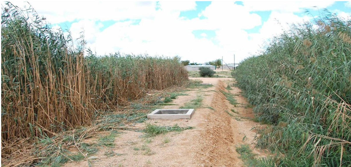
Figure 5 Triple D horizontal flow reedbed WWTWs
