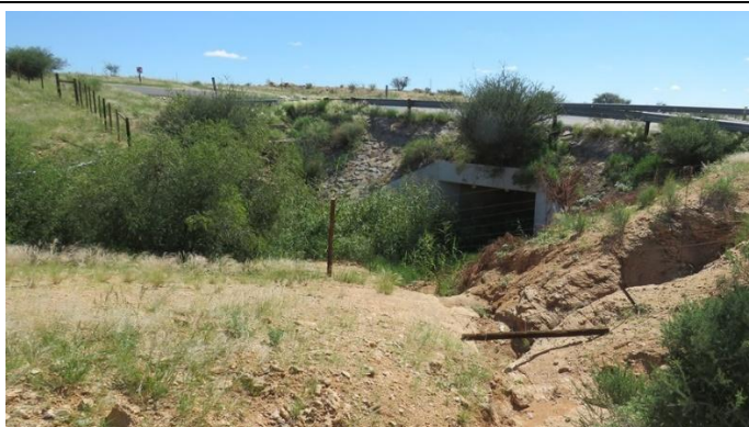
Photo 6: Photo of the gravity line site culvert running under N14
