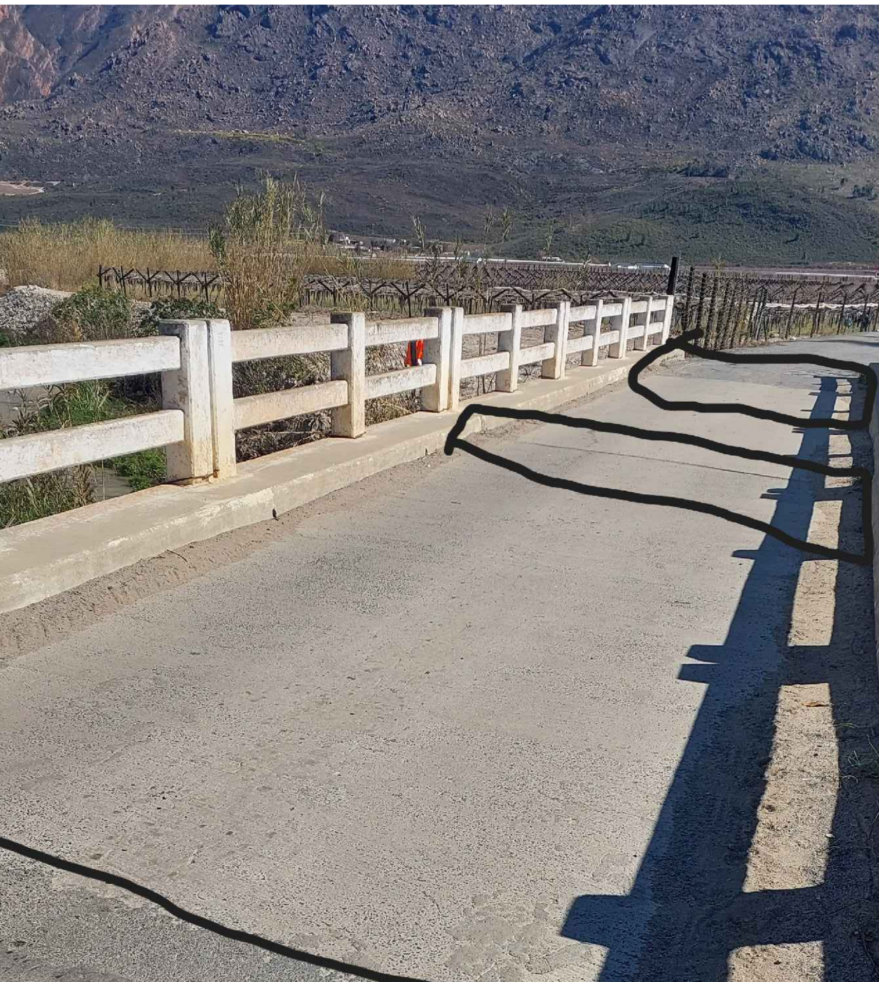
PHOTO 3: SERVICE AND REPAIR OF BRIDGE JOINTS
