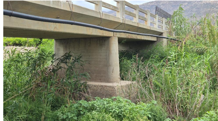
Photo 6: View of Bridge 0496 showing Pier 1 footing of the bridge for which gabion basket installation is proposed to give protection from further erosion
