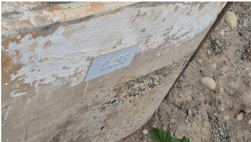
Photo 7: Close-up view showing labelling of Bridge 0496.
