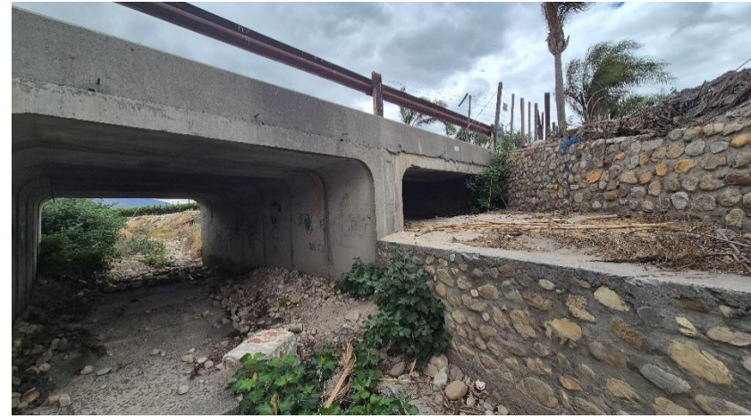
Photo 2: Photograph of Culvert C10432 of existing gabion basket (facing downstream)
