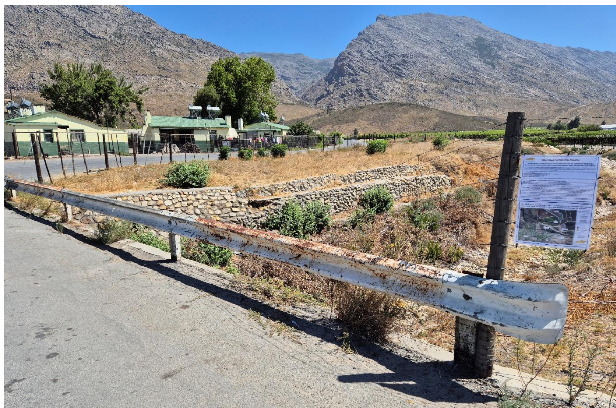
Photo 2: View from further away of the site notice placed at Culvert 10432
