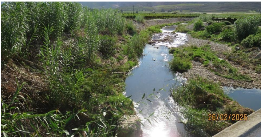
Photo 4: Hex River. The outlet (western side) of the bridge over the Hex River. .
