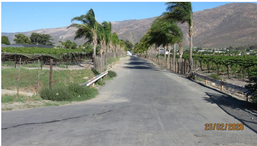
Photo 2: Looking from end of the road west towards the farmhouses in the background (the railings of Culvert 10432 can be seen in the foreground). Note the transformed status of the site.
