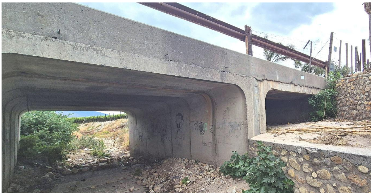
Figure 7 Rooielskloof River Culvert 10432 (Photo Enviro Africa)
