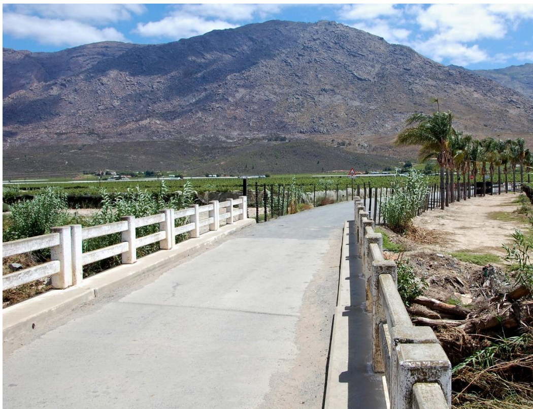
Figure 6 Bridge 0496 over the Hex River at De Doorns
