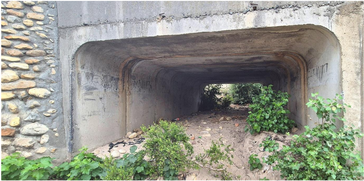
Figure 11 Rooielskloof River Culvert 10432
