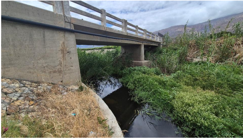
Photo 5: View of Bridge 0496 showing the Hex River flowing underneath
