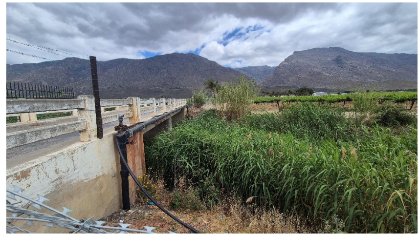
Photo 8: View of Bridge 0496 from the eastern side.
