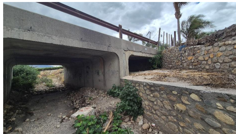
Photo 2: Photograph of Culvert C10432 of existing gabion basket (facing downstream)
