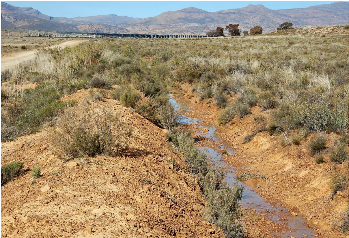
Figure 11 Trench at Drainage Line No. 1.
