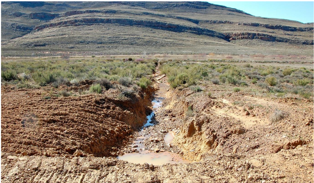
Figure 12 Trench to the river at Drainage Line No.1.
