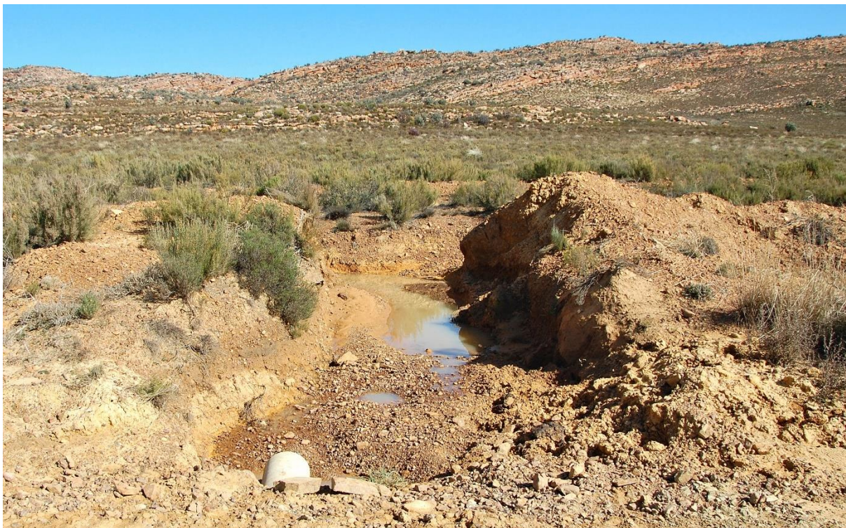
Figure 10 Drainage Line No. 1 pipe culvert.
