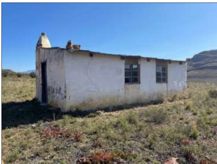
Figure 22. Abandoned farm labourer cottage (waypoint 206). The zinc roof & steel windows have been replaced. The fire place is also a later addition
