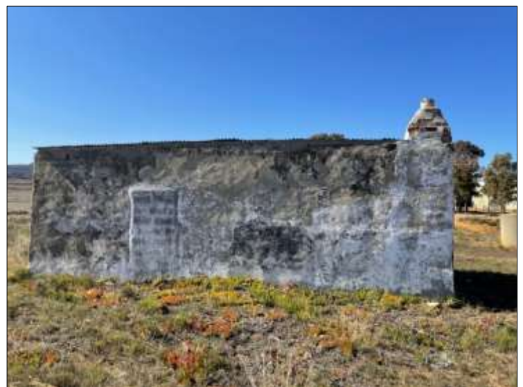
Figure 23. Abandoned farm labourer cottage. Note the back door entrance has been bricked up
