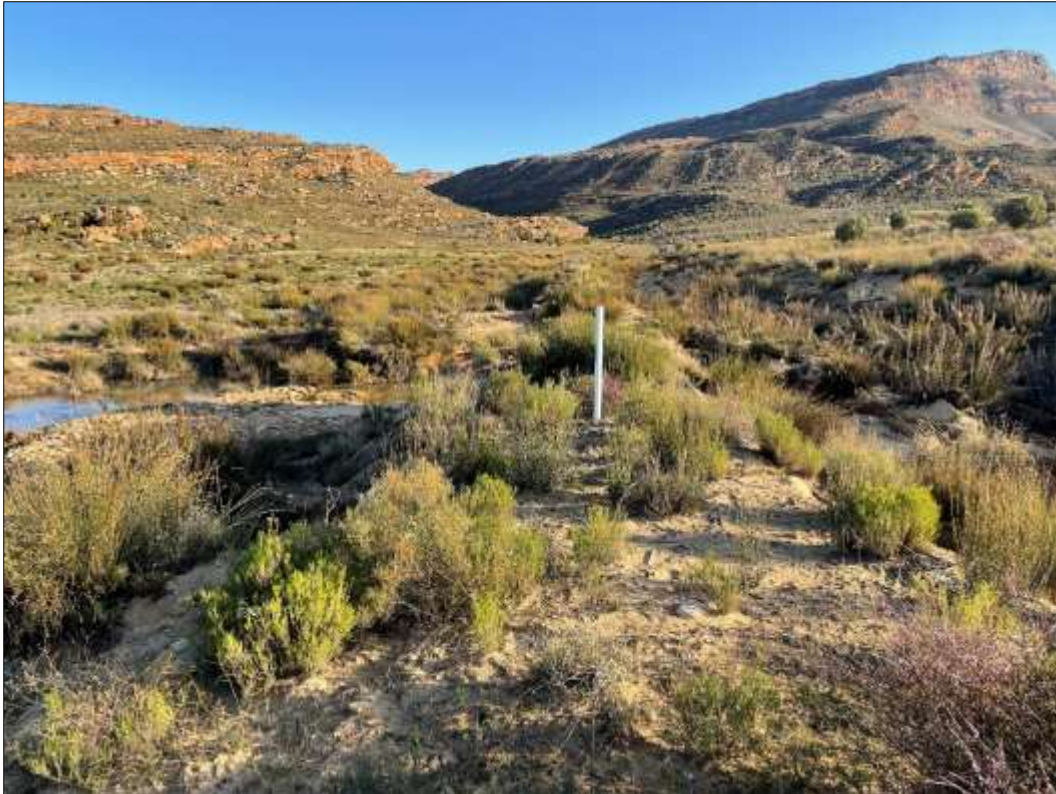
Figure 5. Footprint of the proposed new Harmony Dam. The white pin is the position of the new dam wall. The heritage practitioner is standing on the old dam wall. View facing south (August 2024).
