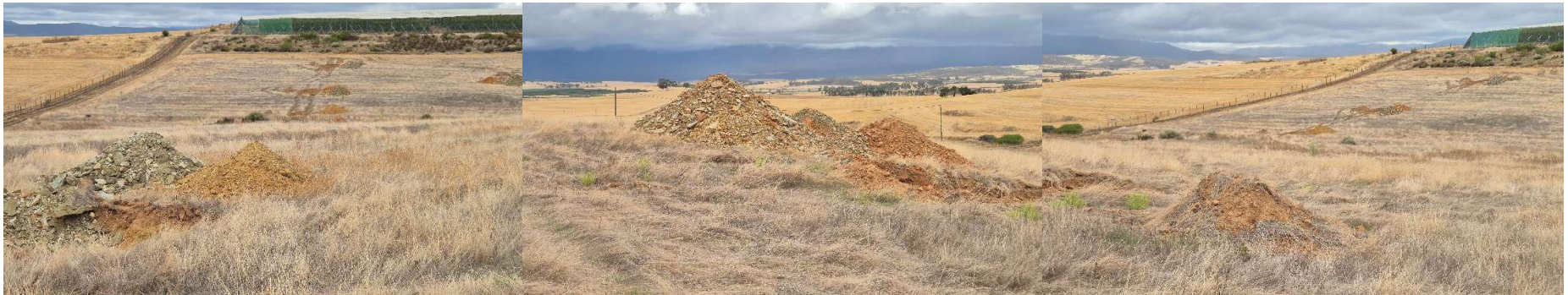
Photo 2: Visible test bits to show where the dam wall is to be located.
