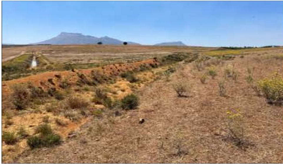
Figure 6: Proposed buffer dam. View facing northwest. Klein Tafelberg can be seen in the distance.
