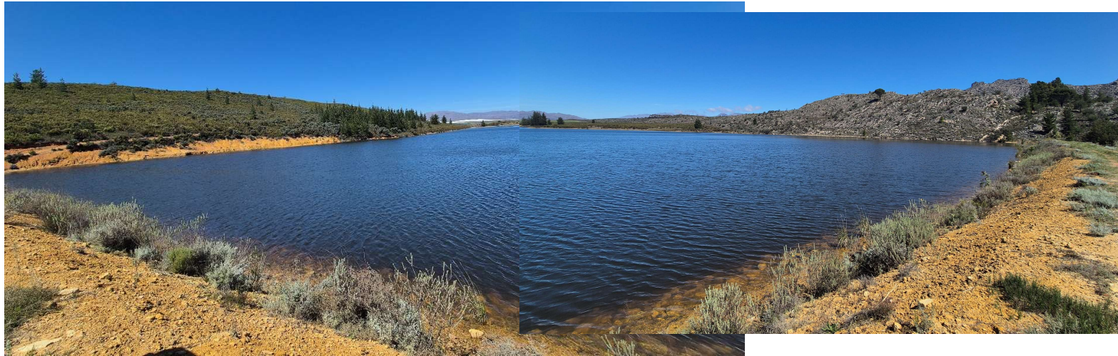
Photo 1: From the northern boundary of existing dam wall looking south (from photo point 3)
