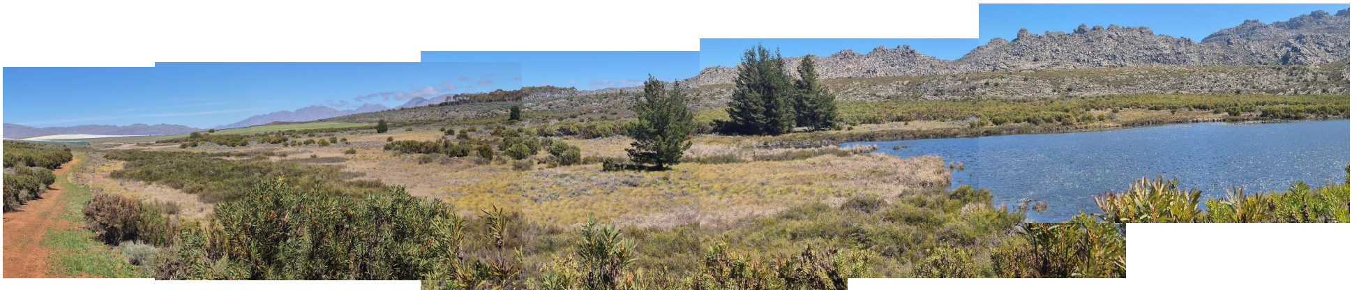
Photo 2: From the eastern boundary, at the end of the existing dam, looking over the proposed new dam extension looking S-W (from photo point 4)
