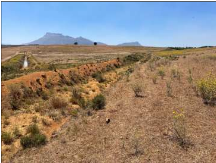
Figure 11. Proposed buffer dam. View facing northwest. Klein Tafelberg can be seen in the distance (November 2025)
