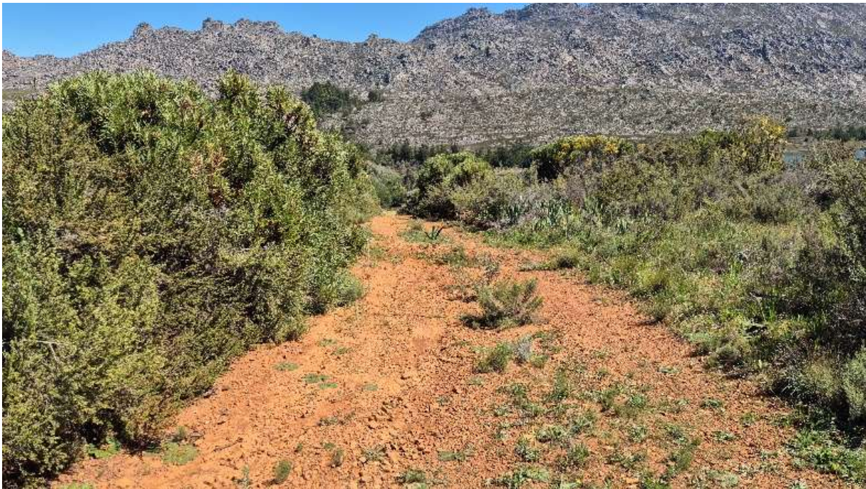
Figure 5. The proposed connecting pipeline looking east towards the existing dam.
